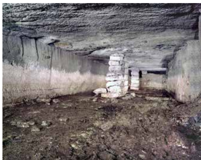
Quarry gallery at Godstone Hill from which spoil has been removed, possibly to make mushroom beds and / or for sale for hearthstone. Note the characteristic smooth walls with arcuate pick marks.
